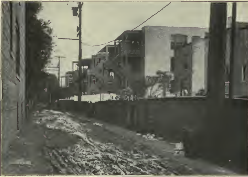
FIG. 37. UNIMPROVED ALLEY. Photograph taken September 4, 1914. A constant stream of delivery, coal, ice and peddlers' wagons passes over the alleys of the city. Only a few of these are improved. When wet they are muddy and unsightly; when dry they are prolific sources of dust.
